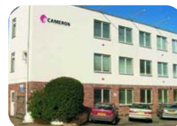
Tunbridge Wells, UK Jiskoot™ Quality Systems Tech Center
